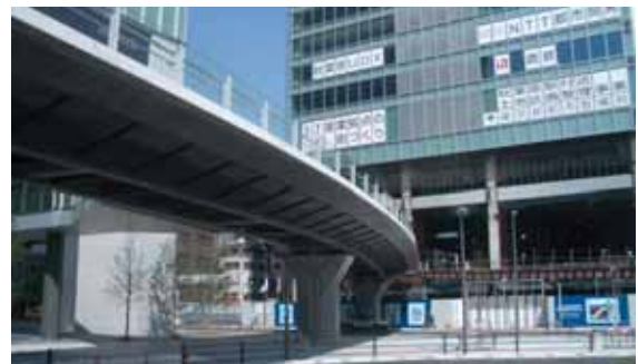
Akiba Bridge ( f'_{ck}=120\text{N/mm}^2 )
