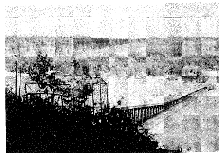
写真— 2.63 Food Canal Bridge (完成)
