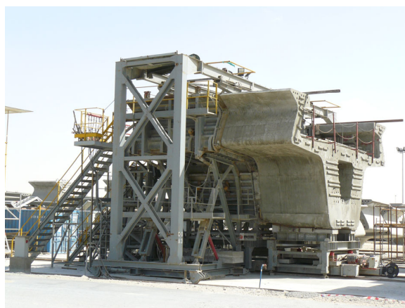
写真-2 C3A型枠
