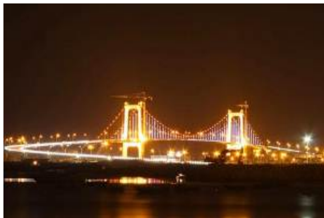
Fig. 7 Thuan Phuoc Bridge
