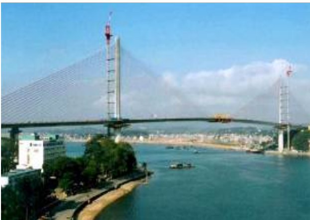
Fig. 4 Bai Chay Bridge
