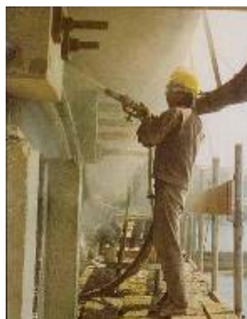
Fig. 13 Repair Y Bridge
