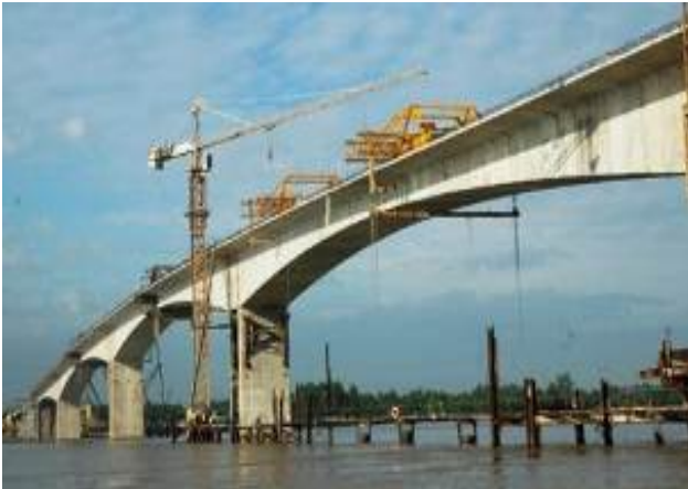
Fig. 10 Ham Luong Bridge
