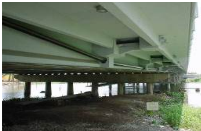
Fig. 17 Strengthening Saigon Bridge
