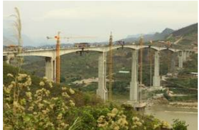
Fig. 11 Pa Uon Bridge
