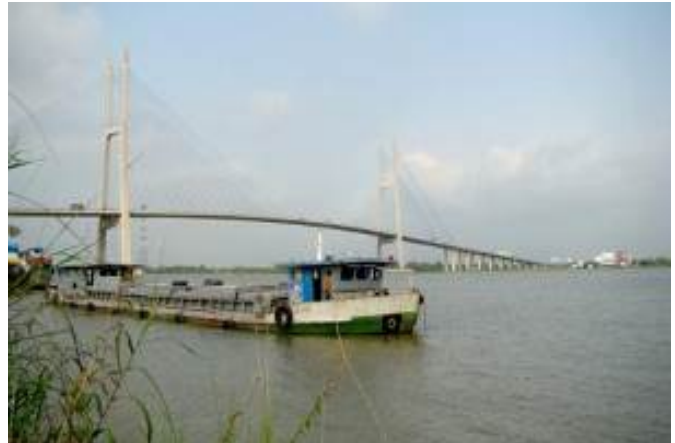
Fig. 3 Rach Mieu Bridge
