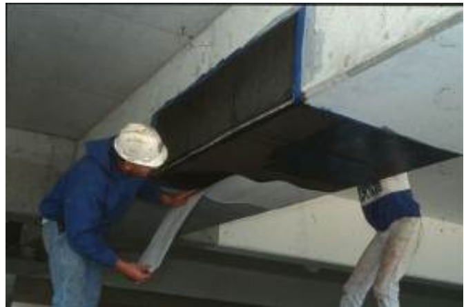
Fig. 15 Strengthening by FPT Material
