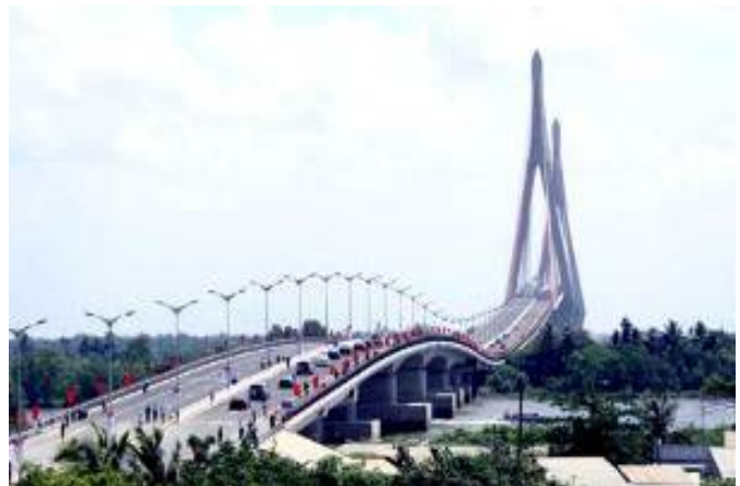
Fig. 5 Can Tho Bridge
