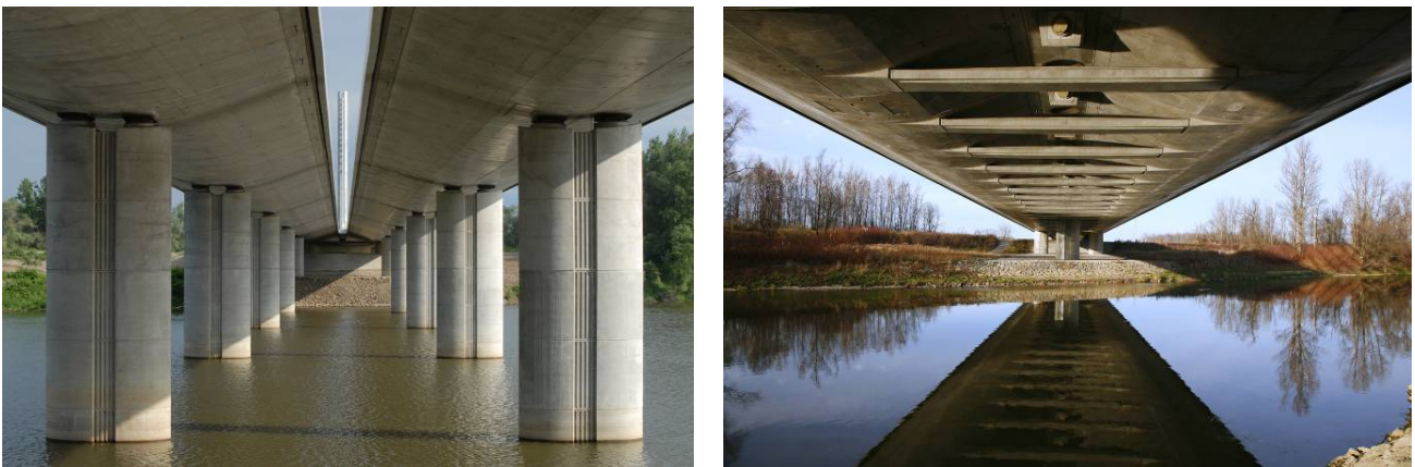
Fig. 9 – Bridge across the Odra River and Antosovice Lake
