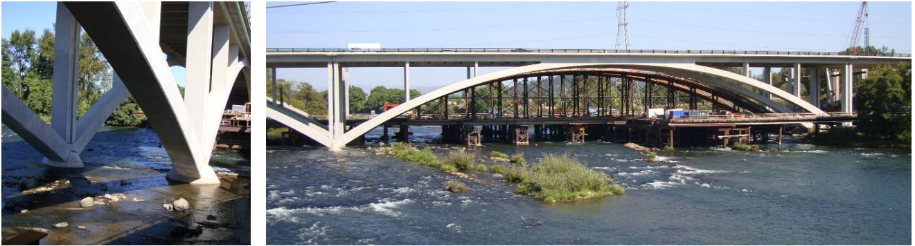
Fig. 6 - Willamette River Bridge, Eugene
