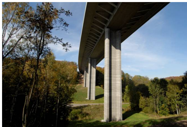
Fig. 3 - Bridge across the Rybny Potok
