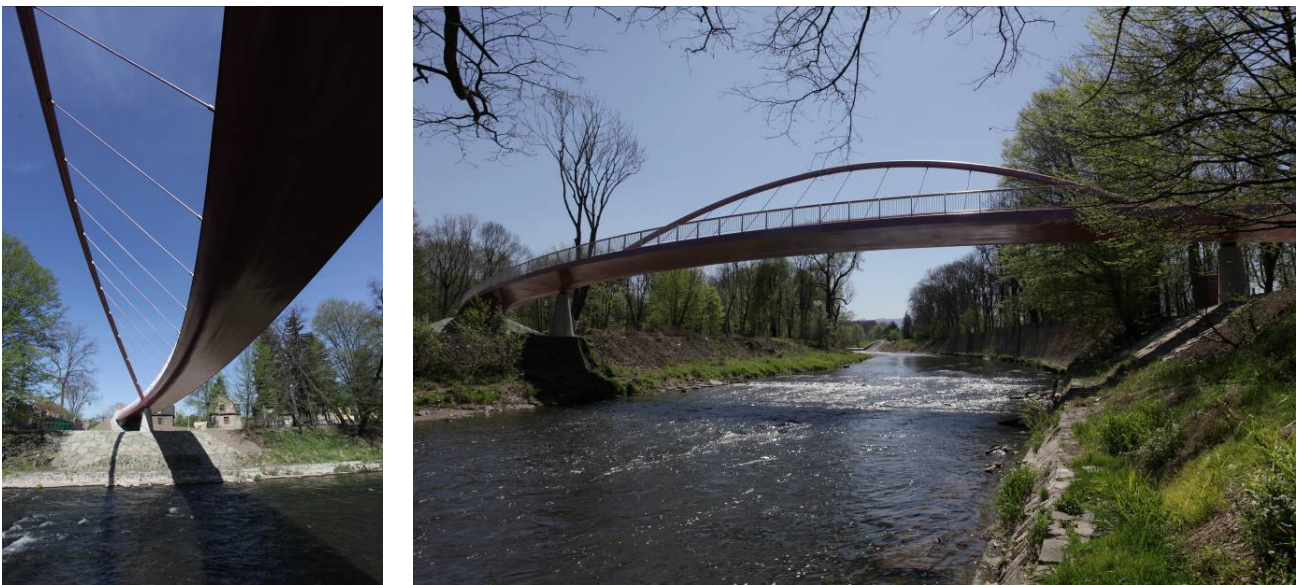
Fig. 13 - Pedestrian Bridge across the border River Olse
