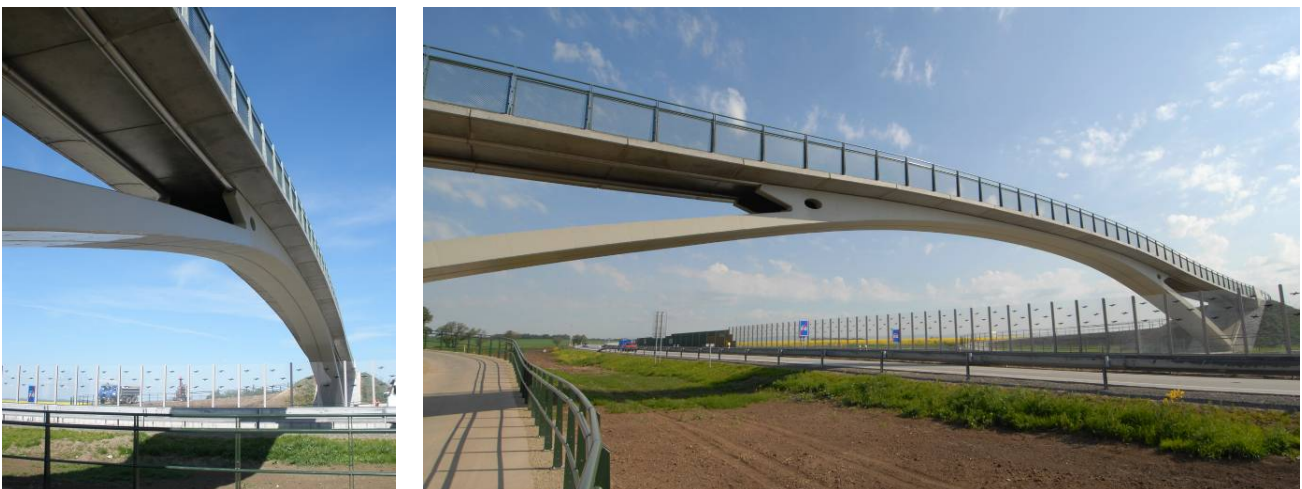
Fig. 15 - Bridge across the expressway R3508 near Olomouc
