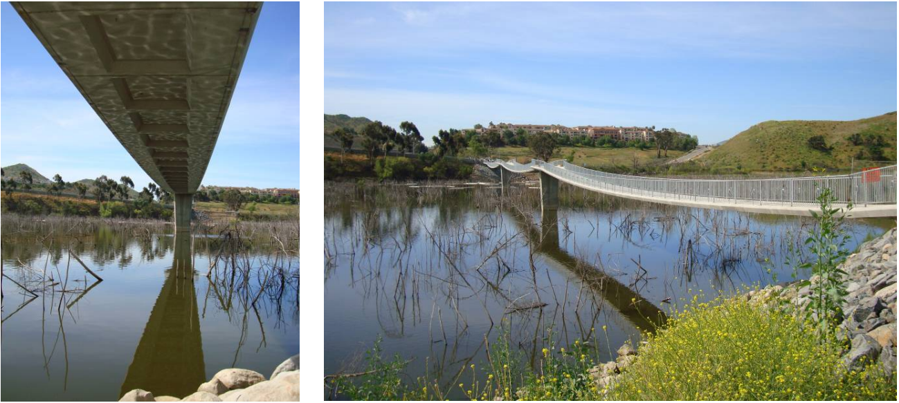
Fig. 14 - The Lake Hodges Bridge, San Diego, California
