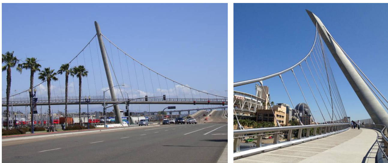
Fig. 12 - Harbor Drive Bridge, San Diego, California
