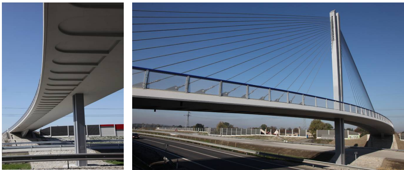
Fig. 11 - Bridge across the freeway D1
