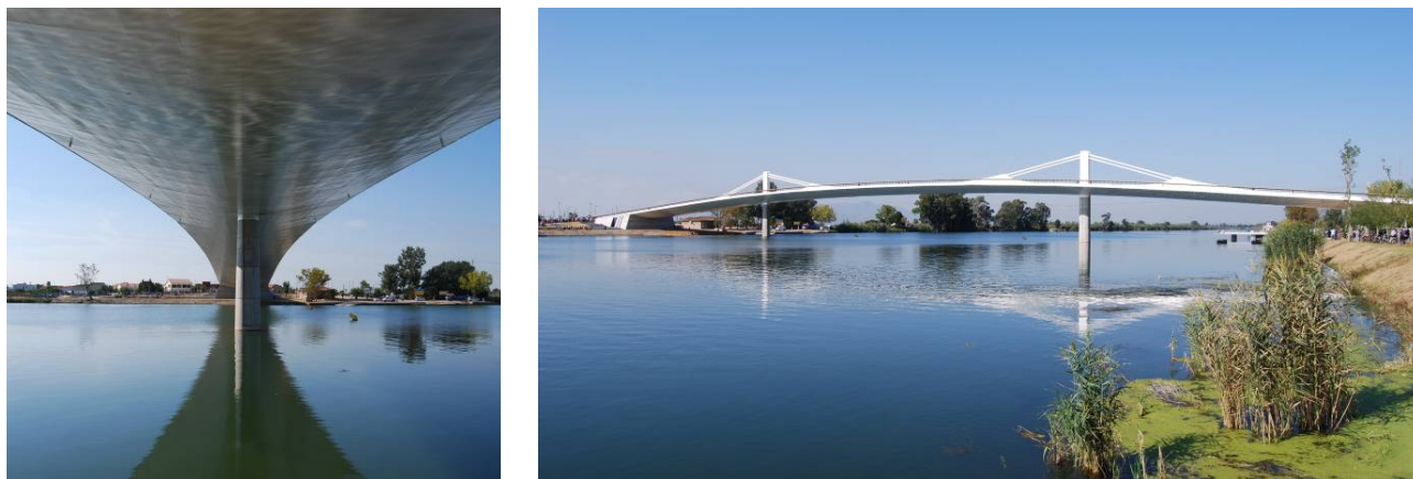
Fig. 10 - Bridge across the River Ebro, Spain
