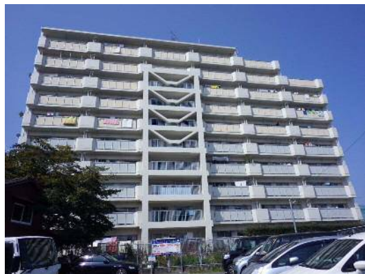
写真-7 補強後外観 (B棟)
