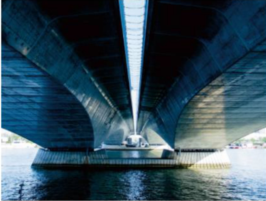
Ryuta Ohashi Bridge
