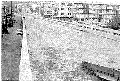
Fig. 19 General view of deck surface
