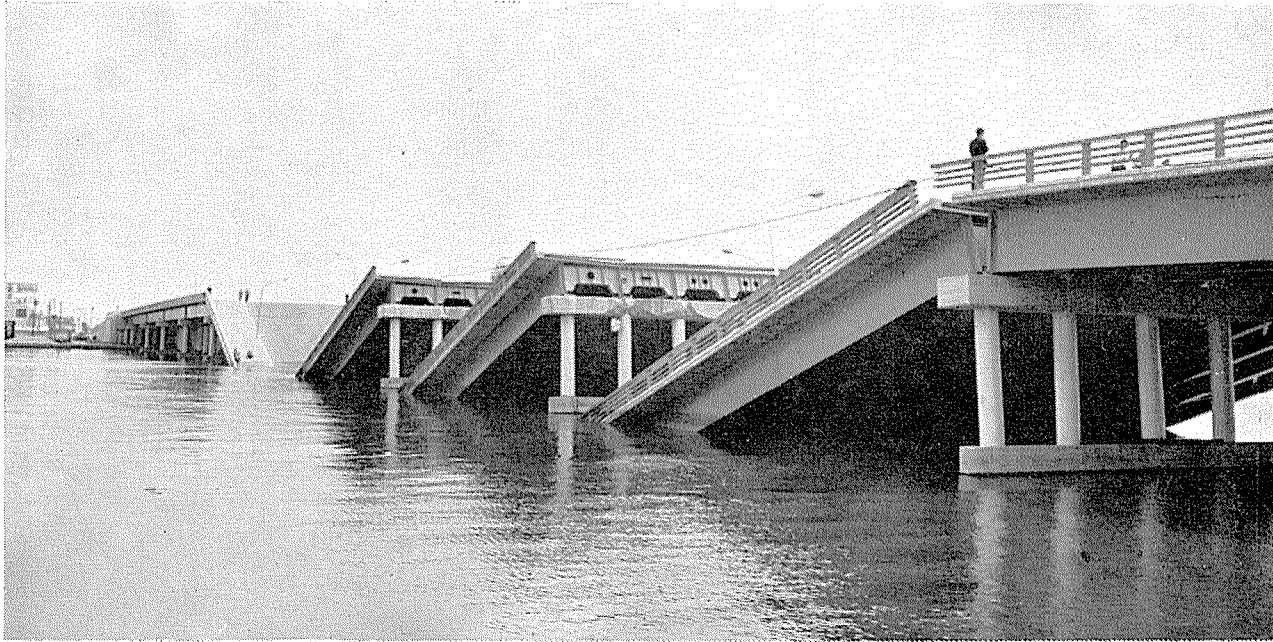
Fig. 4 Steel bridge fell into the Shinano River (Shin-Showa Bridge)
