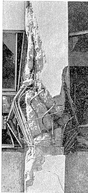
Fig. 8 Breaking up of tie bars and buckling of longitudinal bars, Concrete crumbled.
