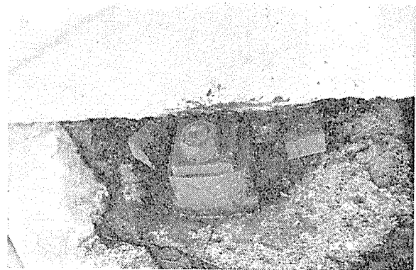
Fig. 17 (b) Tear-off of concrete (Ebino-Earthquake)
