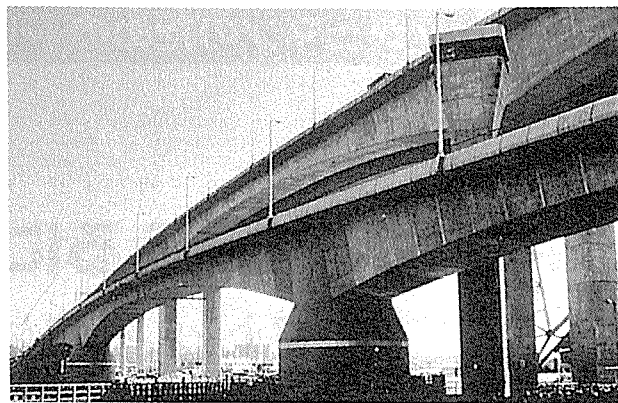
West Seattle Swing Bridge
