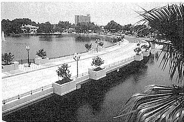
Rasalind Avenue Bridge
