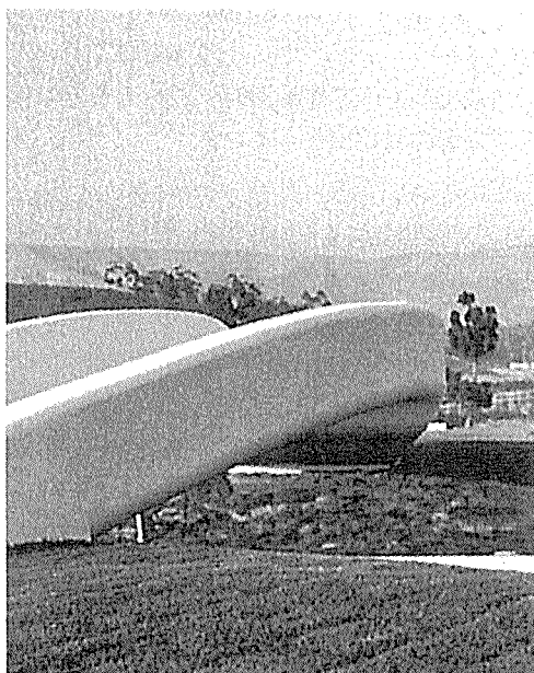
Tustin Ranch Golf Club Entry Bridge
