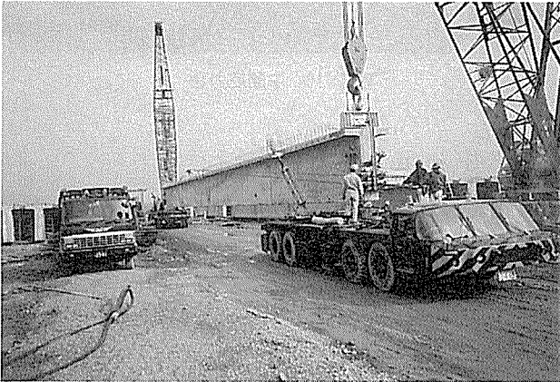
写真-2 桁積込
