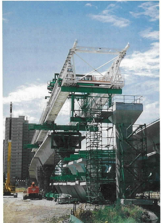
写真-4 Overhead Truss
