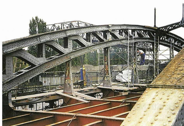
Fig. 7 Stubenrauchbrücke Crossing River Spree in Berlin during Repair Work 1998
