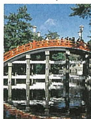
Sorji-bridge at Sumiyoshi Grand Shrine
