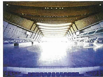
Nagano Olympic Memorial Arena
