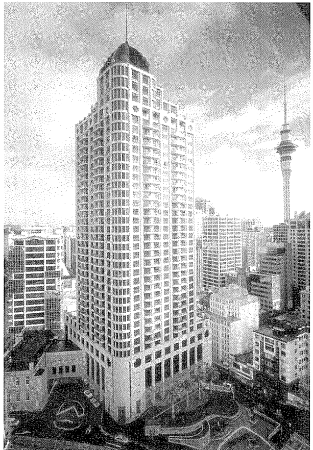
写真 - 1 The Metropolis Regency (Courtesy of Holmes Consulting Group, Structural Engineers)
