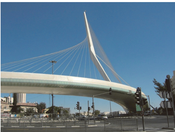
写真 - 13 Jerusalem Chords Bridge (写真: Little Savage)
