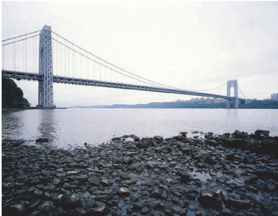
写真 - 3 George Washington Bridge, USA. Design: Othmar Ammann
