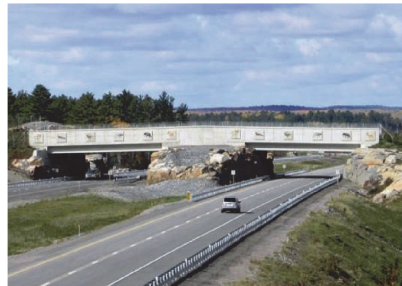
写真 - 5 Wildlife Overpass, Canada. (Source of image: Ministry of Transportation of Ontario)
