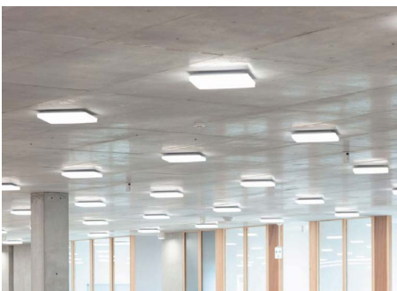
Fig. 6 Interior view of first-floor ceiling without ceiling material
