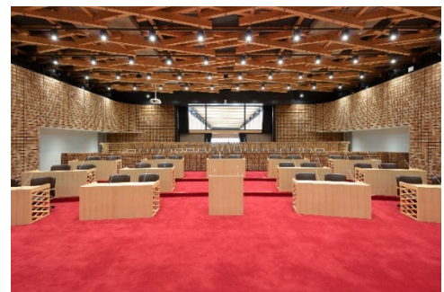
Fig. 8 Wood beams structural system (above); interior view of assembly hall using wood beams (below)
