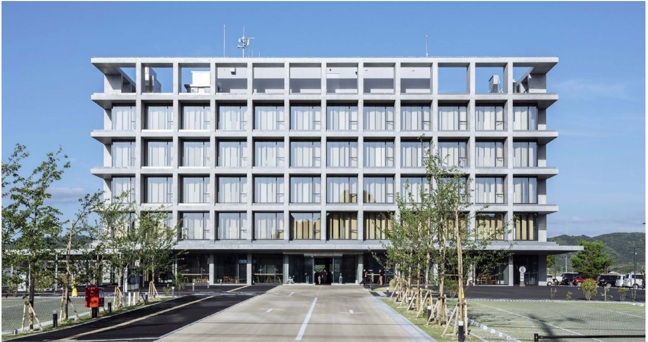
Fig. 2 View from the west
