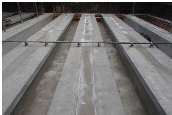
6) Concrete construction on the upper slabs
