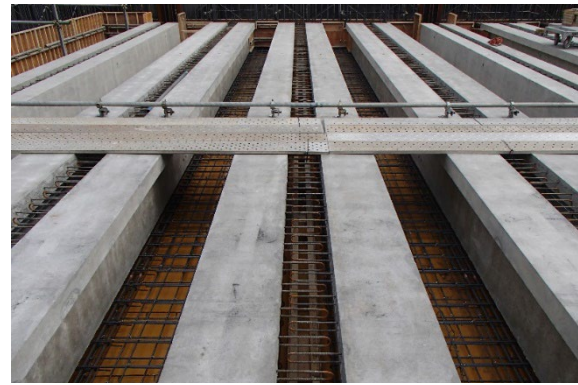
4) Lower slab upper reinforcement
