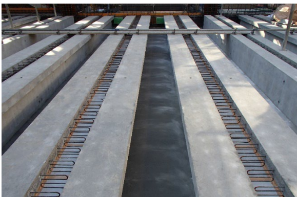
5) Concrete construction on the lower slabs
