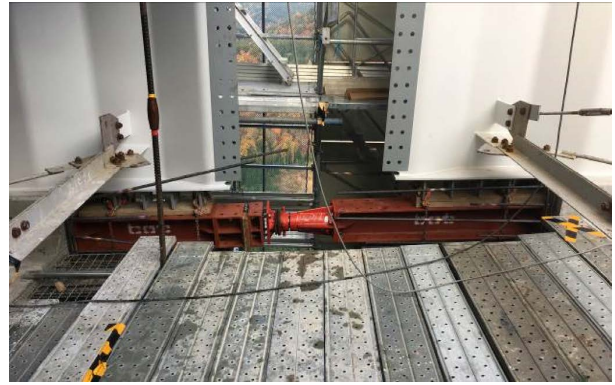
Fig. 10 Horizontal jack to widen the closure
