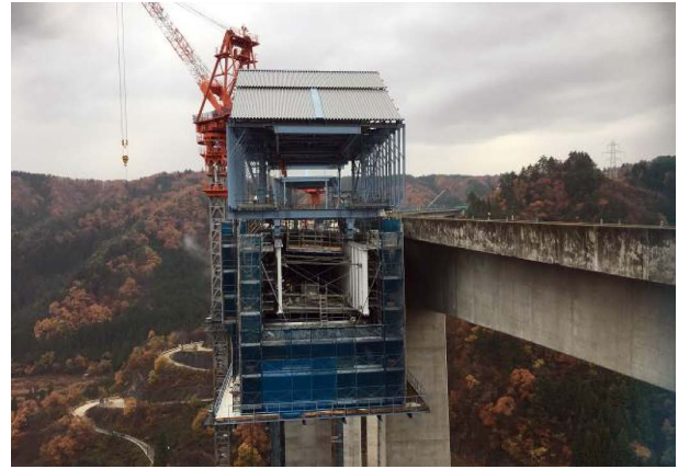
Fig. 8 Form traveller for P1 cantilever
