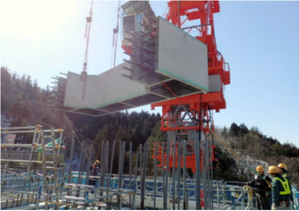
Fig. 6 Installing precast member
