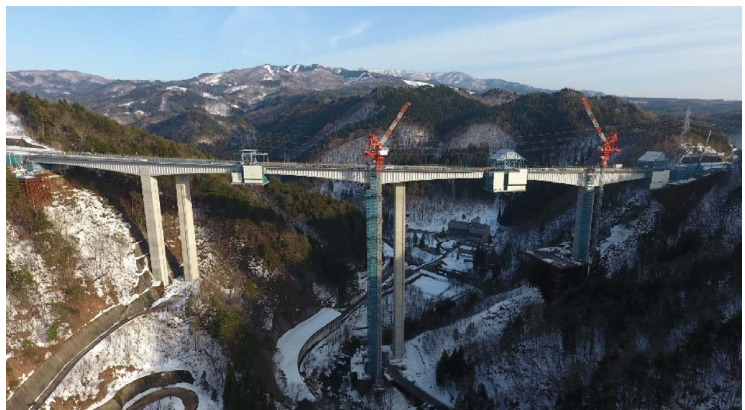
Fig. 11 Washimi bridge (under construction)
