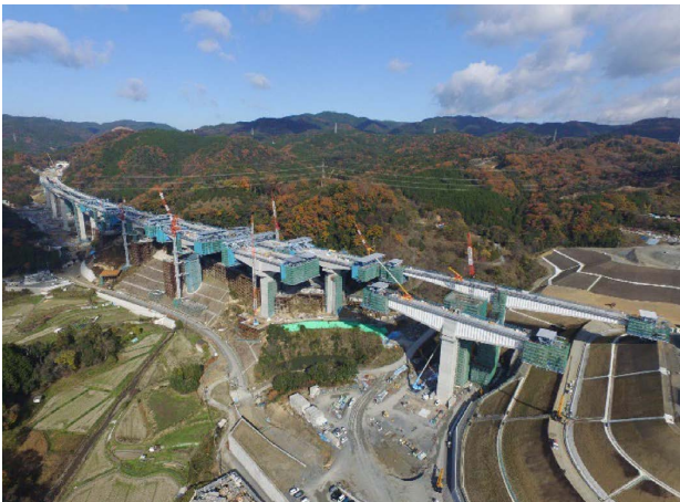
Fig. 4 Cantilever erection at multiple piers
