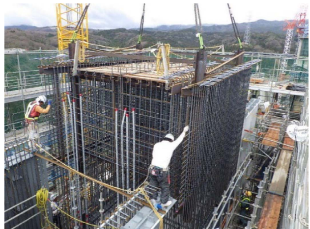
Fig. 7 Erection of prefabricated reinforcement
