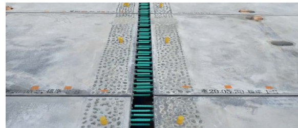
Fig. 6 Longitudinal joint before filling with UHPFRC
